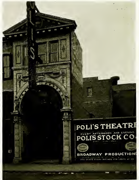
Entrance to Poli Theatre South Main Street
